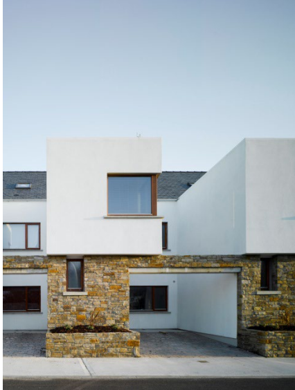
Horizontally coursed 215mm min thickness natural local stone with a beige / reddish hue, and 450mm high raised stone faced planters at the base and as proposed to front boundaries with railings above
