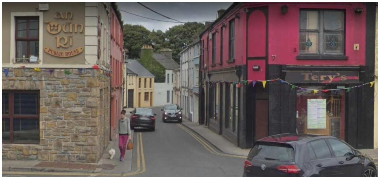
Figure 1.3: Existing Narrow Carriageway
