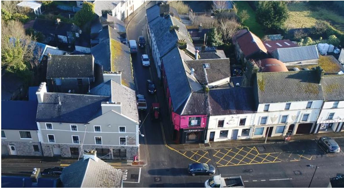
Figure 4.1: Aerial View of Bridge Street, Dunmore
