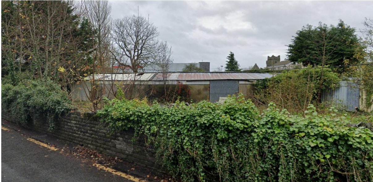
Figure 5.1: Side View of Bridge Street, Dunmore showing Units 9 & 10
