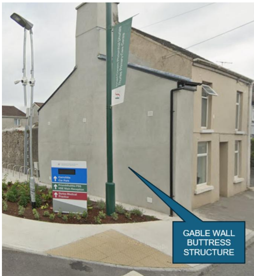
Figure 4.2: Gable Wall Buttress Structure, Dunmore
