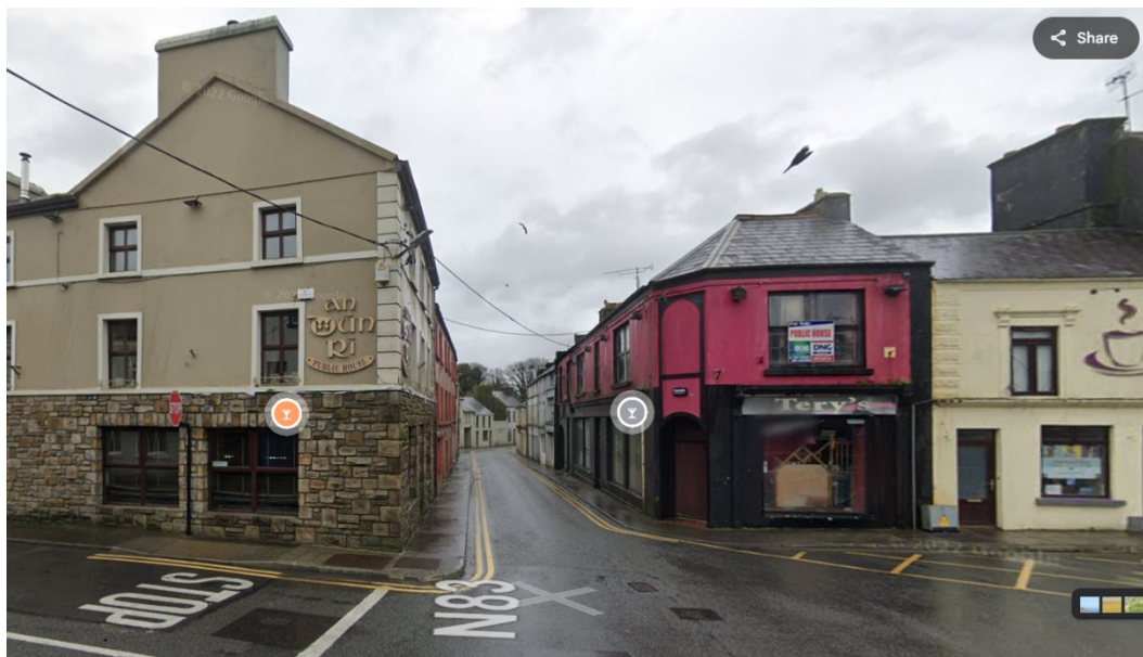
View of Bridge Street in 2022.
