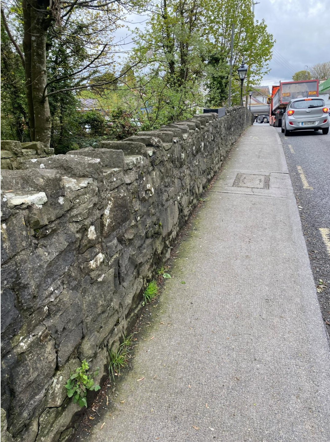
Figure 5.4: Stone bridge (BL1) located north of the site.
