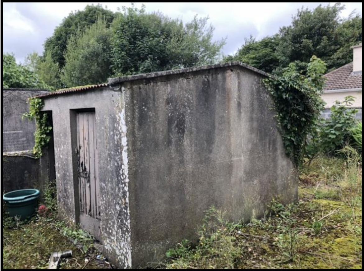
Plate 4.3 Looking west at the shed no.1 on site
