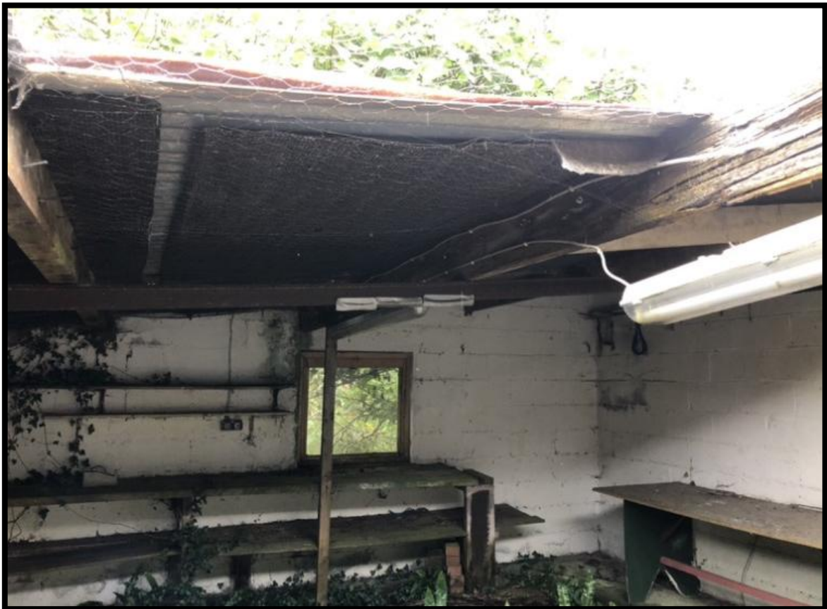
Plate 4.8 Image of the interior of shed no.3 on site
