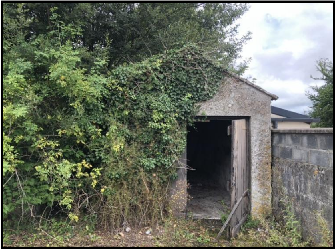
Plate 4.5 Looking west at the shed no.2 on site
