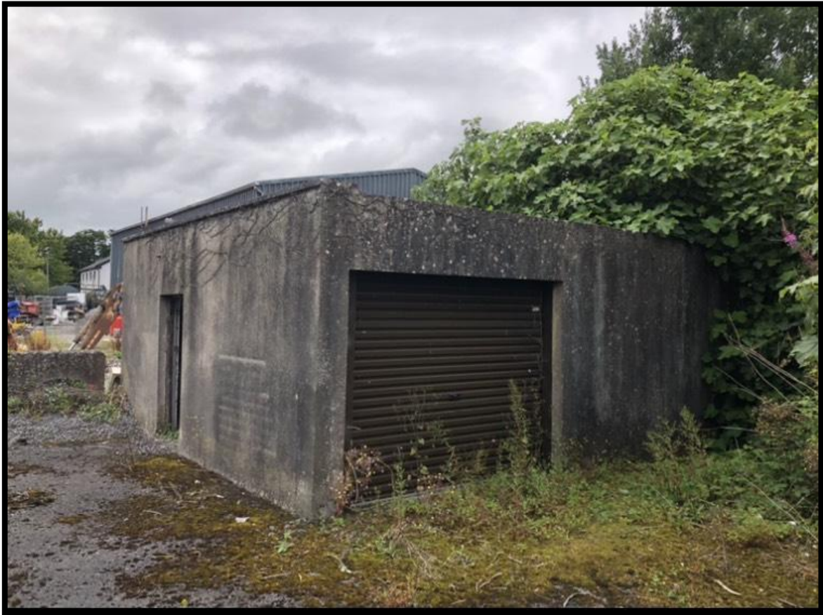
Plate 4.7 Looking south at the shed no.3 on site
