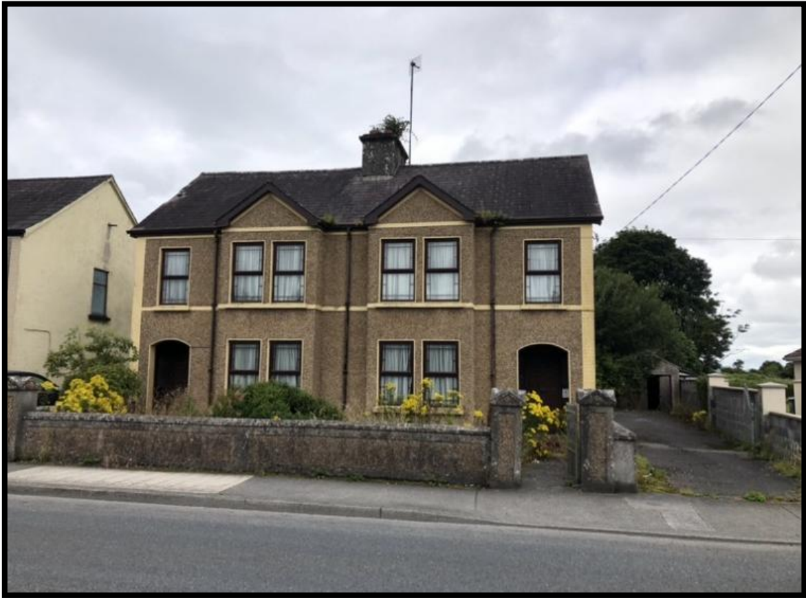
Plate 4.1 Looking west at the existing building on site
