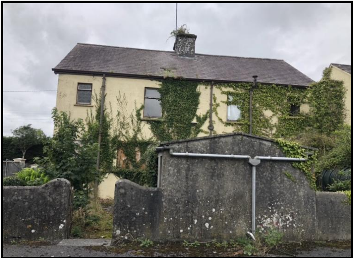
Plate 4.2 Looking east at the rear of the existing building on site
