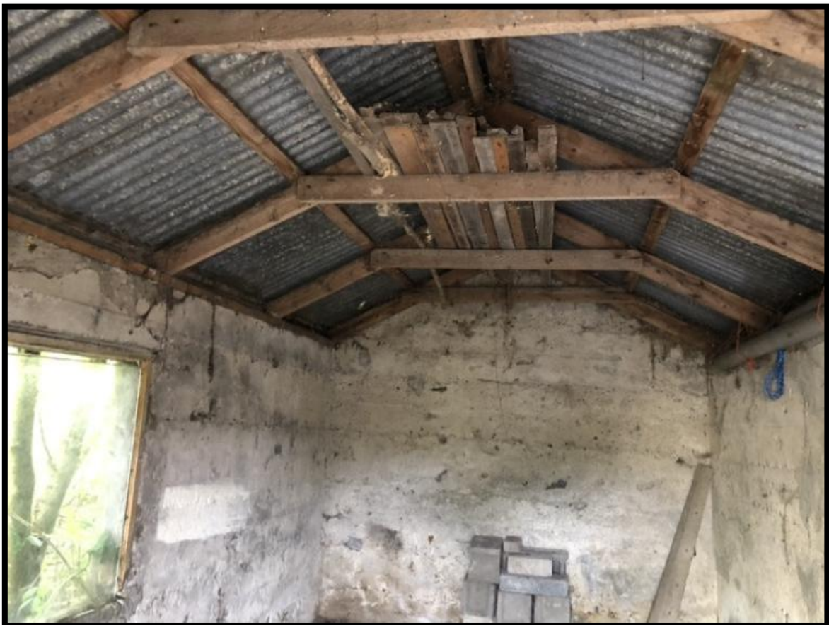
Plate 4.6 Image of the interior of shed no.2 on site
