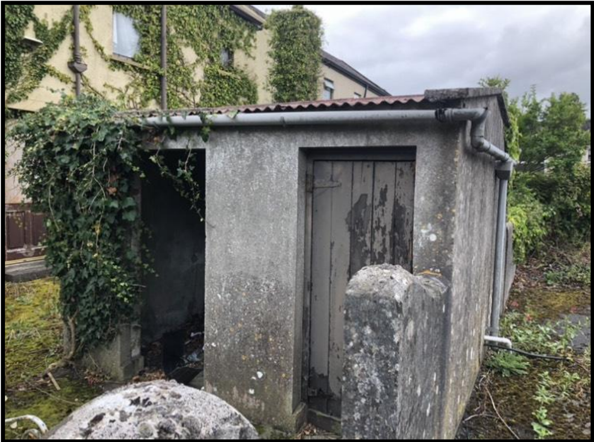
Plate 4.4 Looking south at the shed no.1 on site
