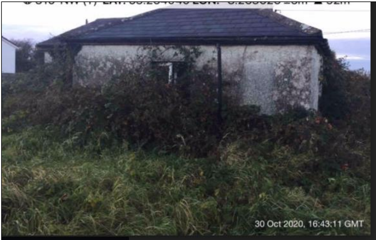
Photographs 3: Photograph taken from within the site
