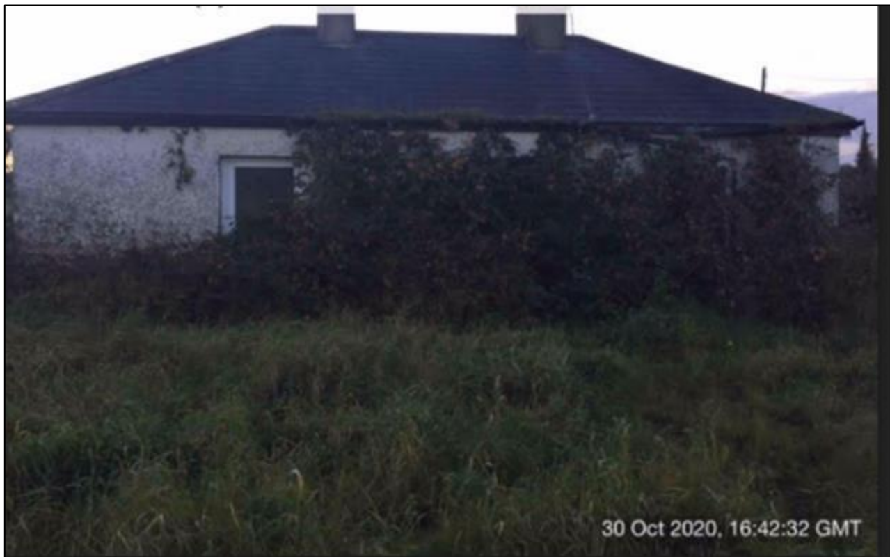
Photograph 1: Front Elevation of The Existing taken from outside the site
