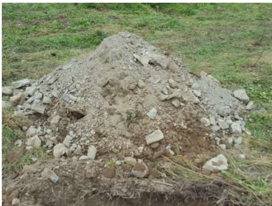
Trial Pit dug to 1.6m deep 29-06-2020.
