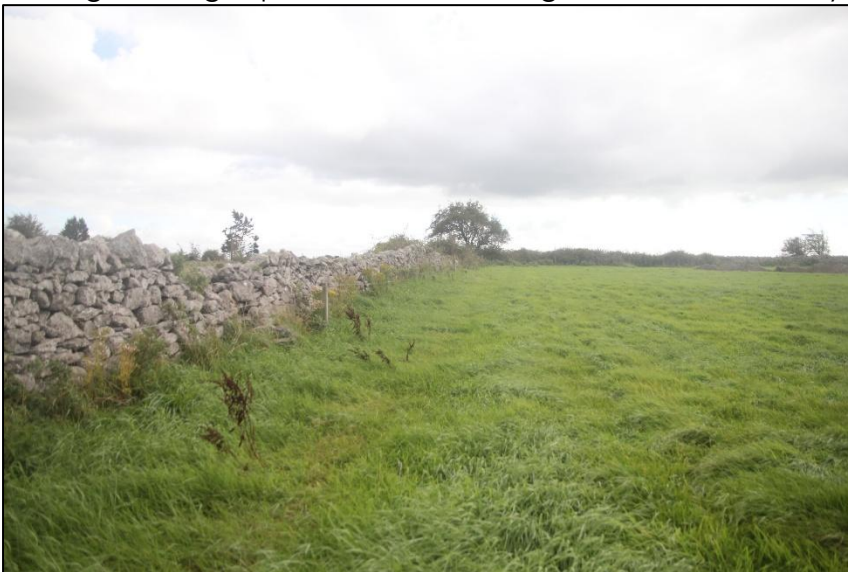
Plate 3: Old stone walls (BL1) forming the eastern site boundary showing typical dry-stone construction.
