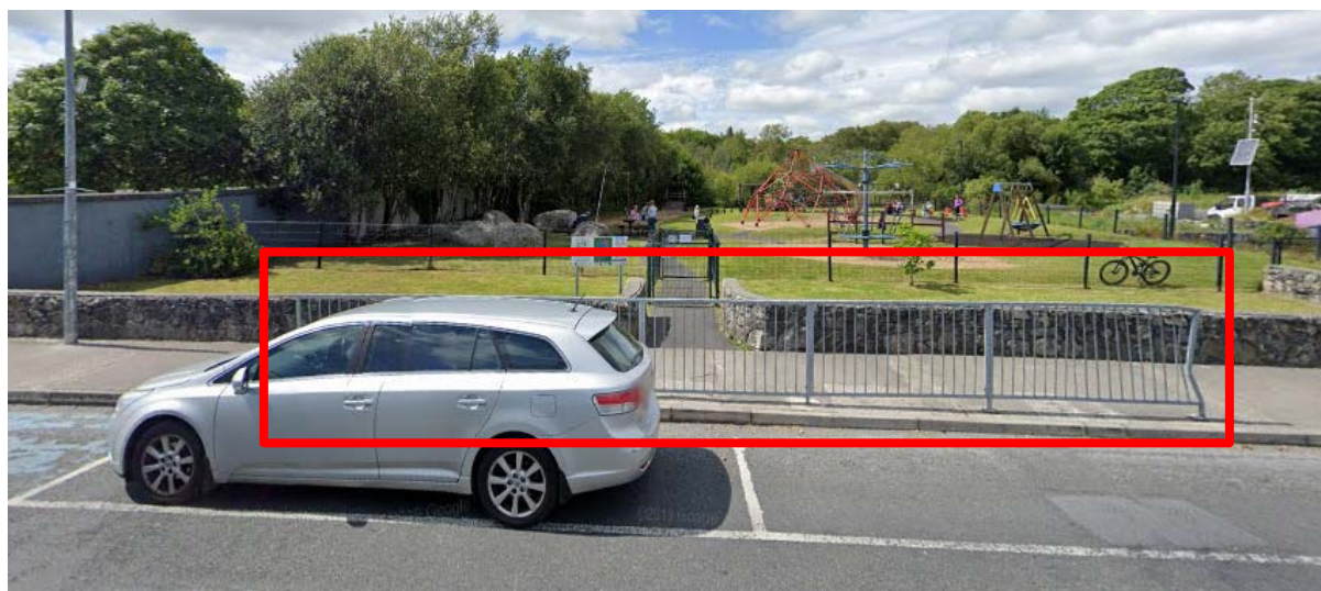
Plate 2-5 L1320 Pedestrian Guardrail adjacent to Playground
