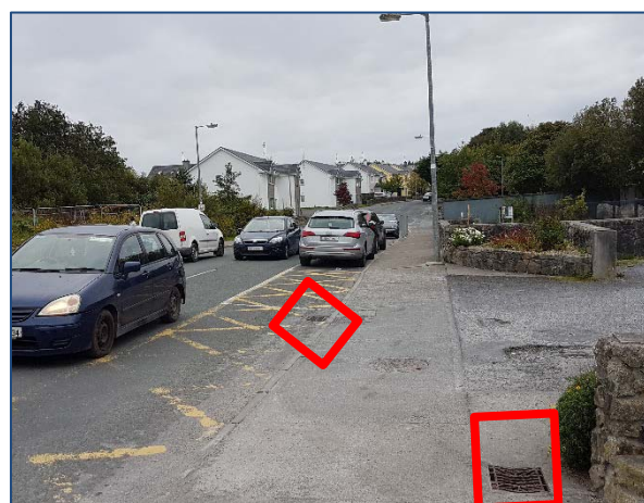
Plate 2-4 L1320 Existing Drainage
