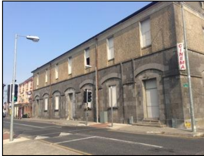
Plate 1: View of building from the SE.
