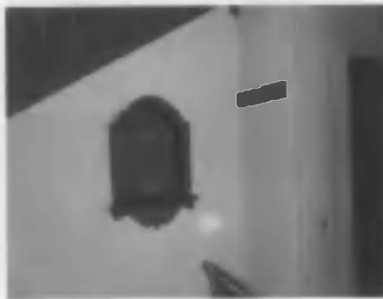
Ticket hatch in main stairwell
