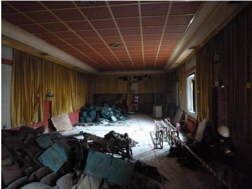
Photo 2. The Cinema with the original seating removed and stacked
