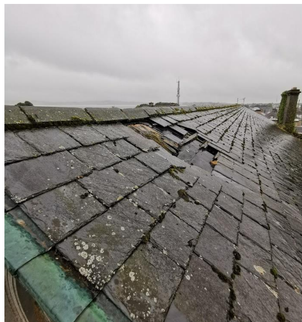
Photo 15 & 16. Lead flashing on the eastern gable and copper flashing of the verges
