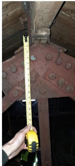
Photo 22, 23 & 24. Rood construction & steel trusses
