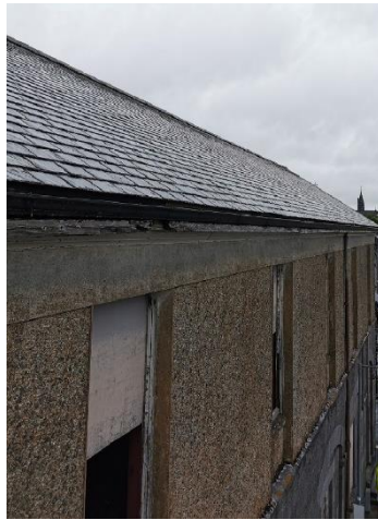
Photo 48. First floor fenestration
