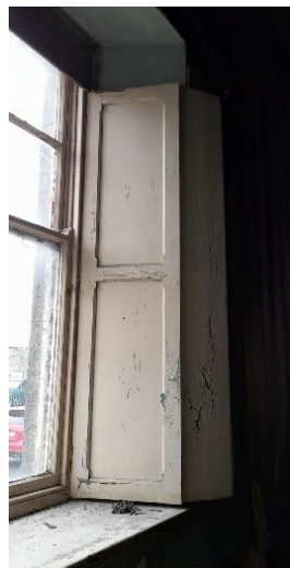
Photo 40. & 41. Ground floor windows
