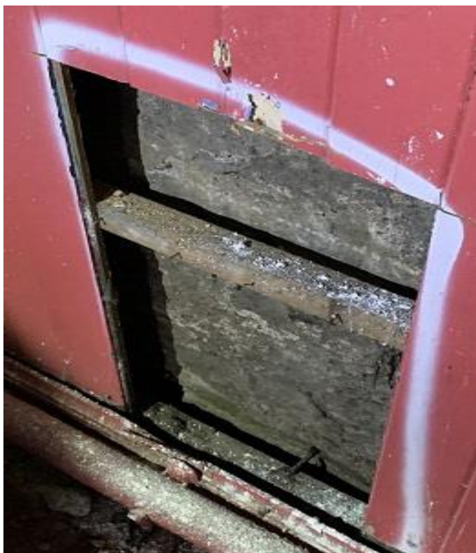
Photo 33. Dry-lining system with timber panelling
