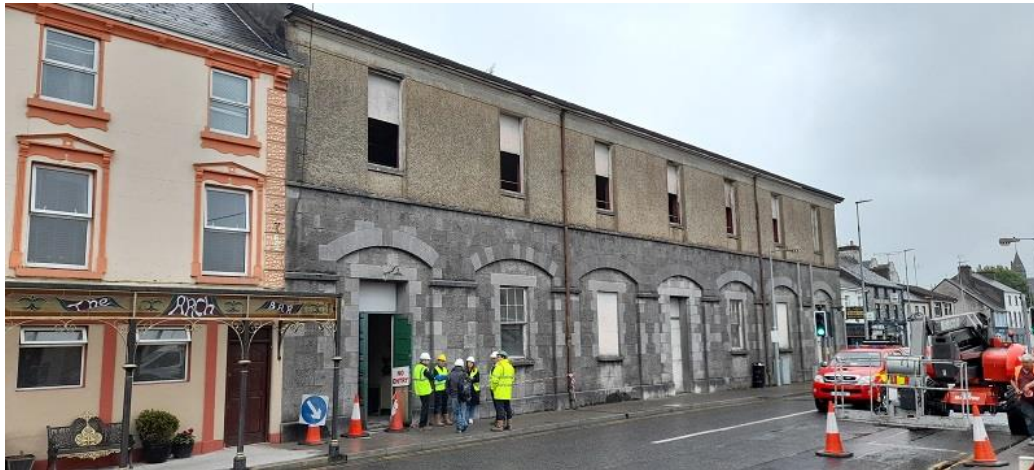
Photo 8. Main building external wall finishes
