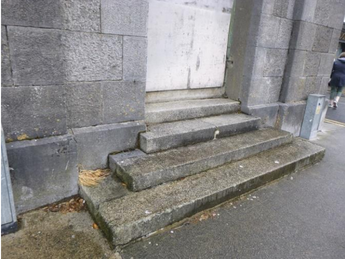
Photo 26. Stone steps at eastern entrance to be removed
