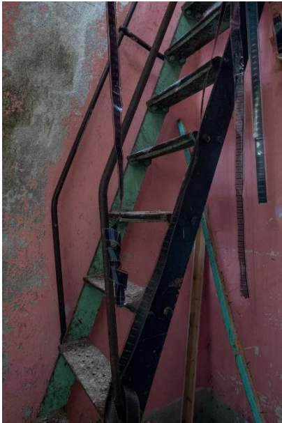
Projector Room photos Photo 27. Metal ladder stairs
