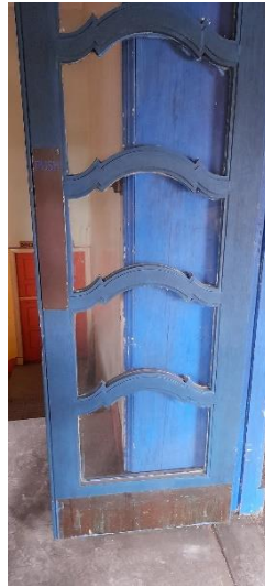
Photo 5 & 6. The Ballroom glazed doors
