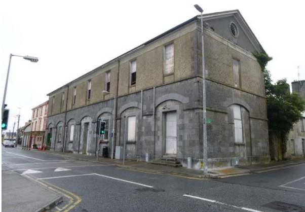
Photo 1. Townhall building in context
