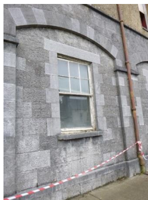
Photo 9 & 10 Main building Ground Floor doors and windows on street elevations
