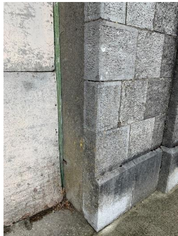
Photo 51. Door opening stonework
