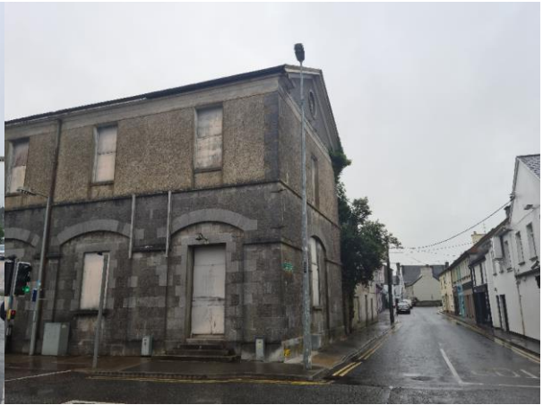
Plate 3-2: Side of building
