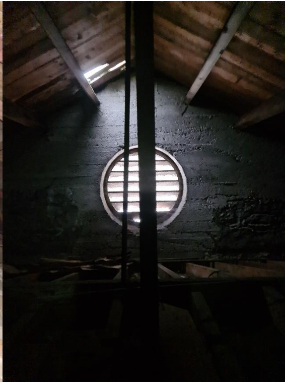
Plate 3-6: Potential entrance point to attic
