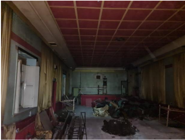
Plate 3-4: Main first floor room
