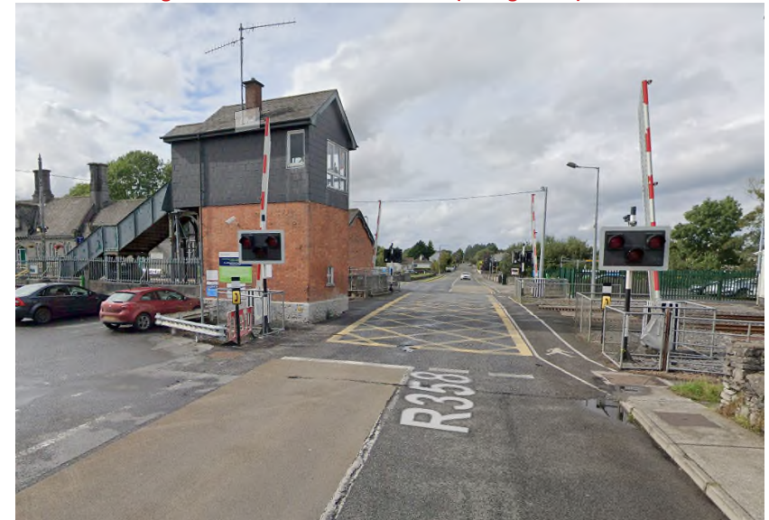
Figure 38. Ballinasloe Station (Facing North)
