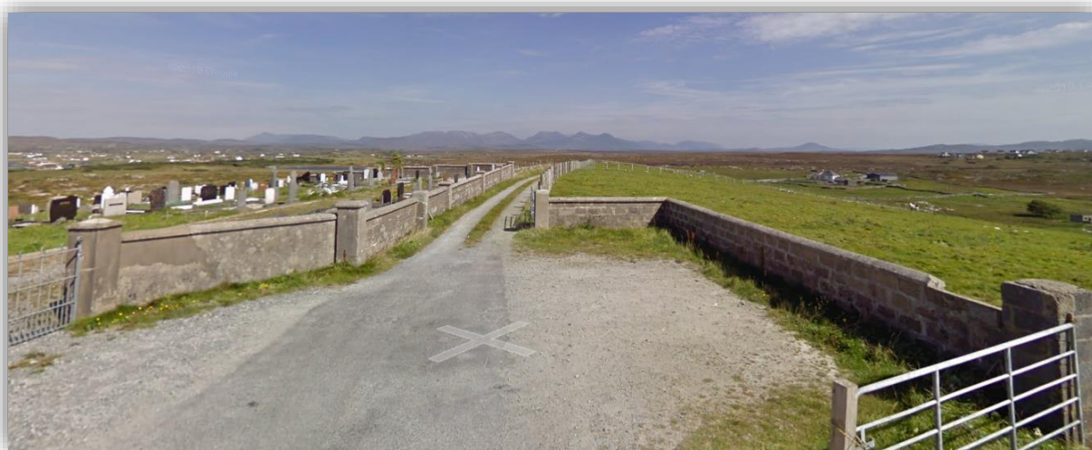
Fig 1 : Entrance & Parking Area
