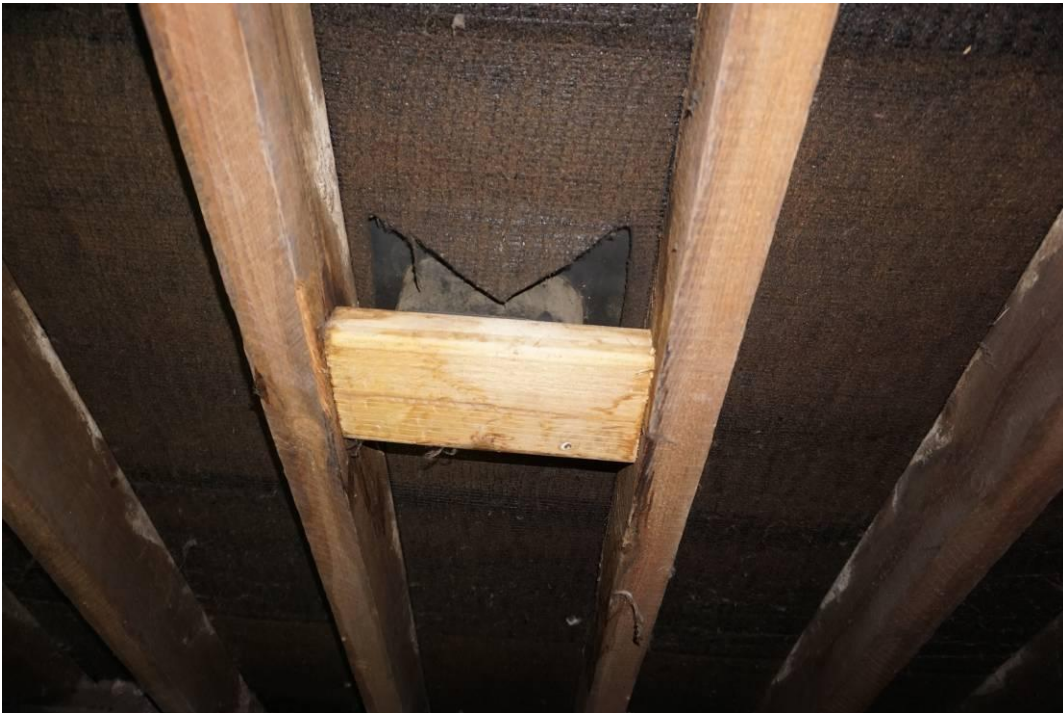
Photograph 28 Attempt to stop water ingress at a slate vent.
