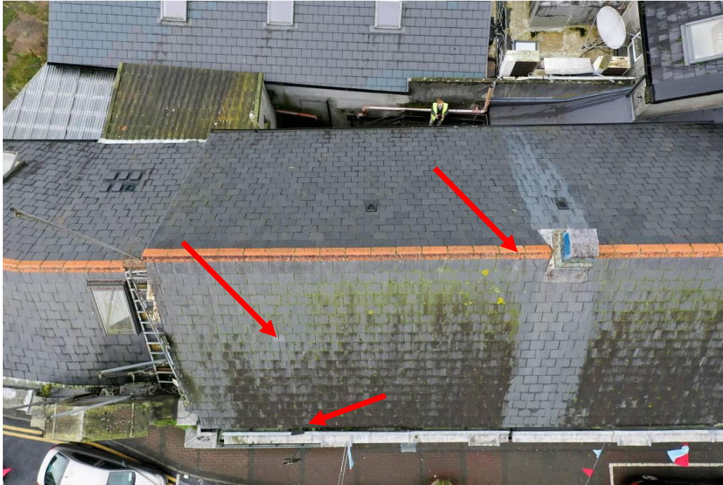
Photograph 21 View of a section of the front roof plane, slipped/failed slates highlighted.
