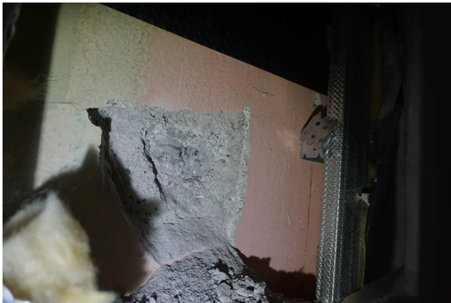
Photograph 38 Opening made to the render, a lime rich cementitious render.
