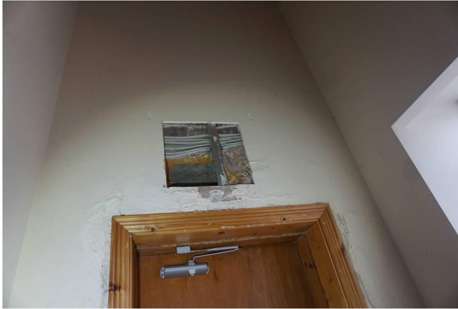
Photograph 22 View of investigative opening up panel. Note cable run.
