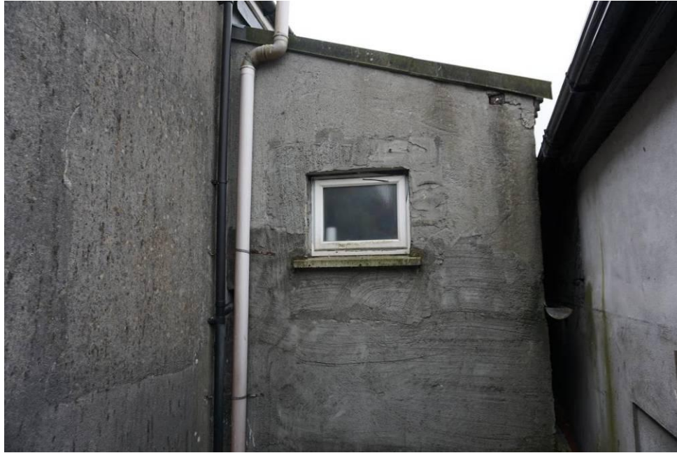
Photograph 14 Patchy render applied to the rear annex.
