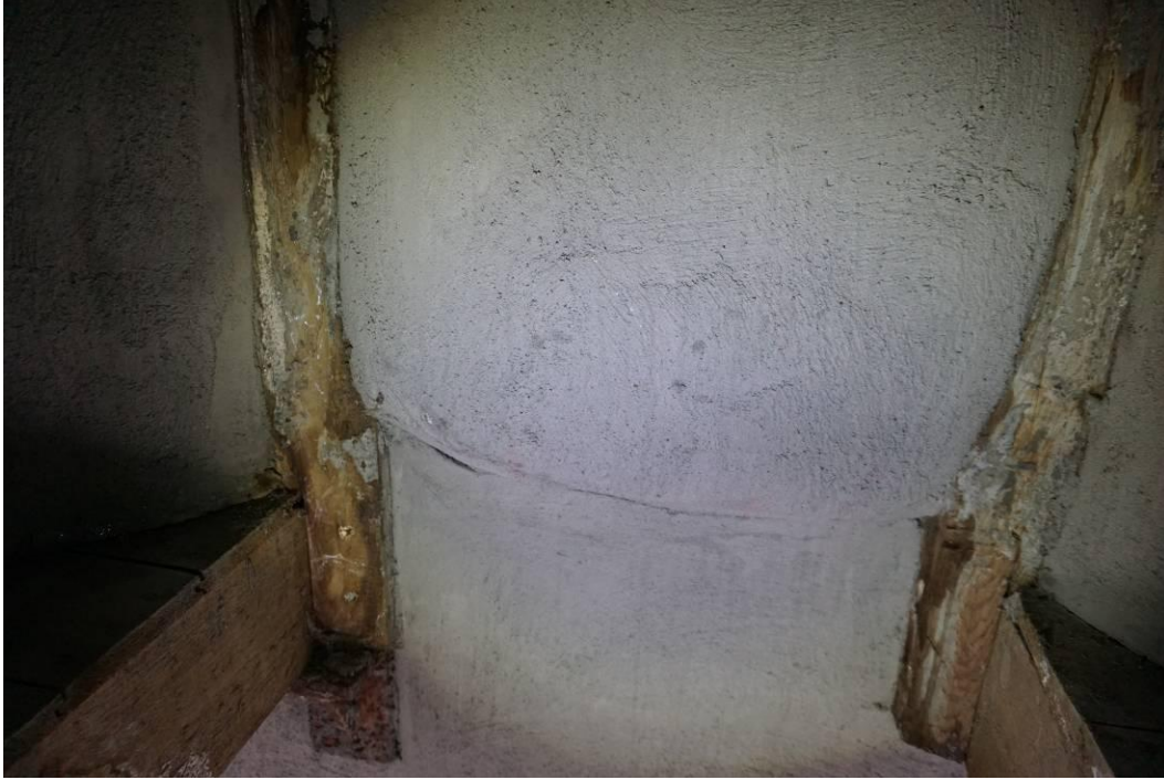
Photograph 4 Example of cementitious rendered panel with crack clearly visible.
