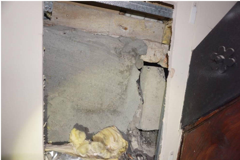
Photograph 32 View of mismatch of materials (off cut of a window cill).
