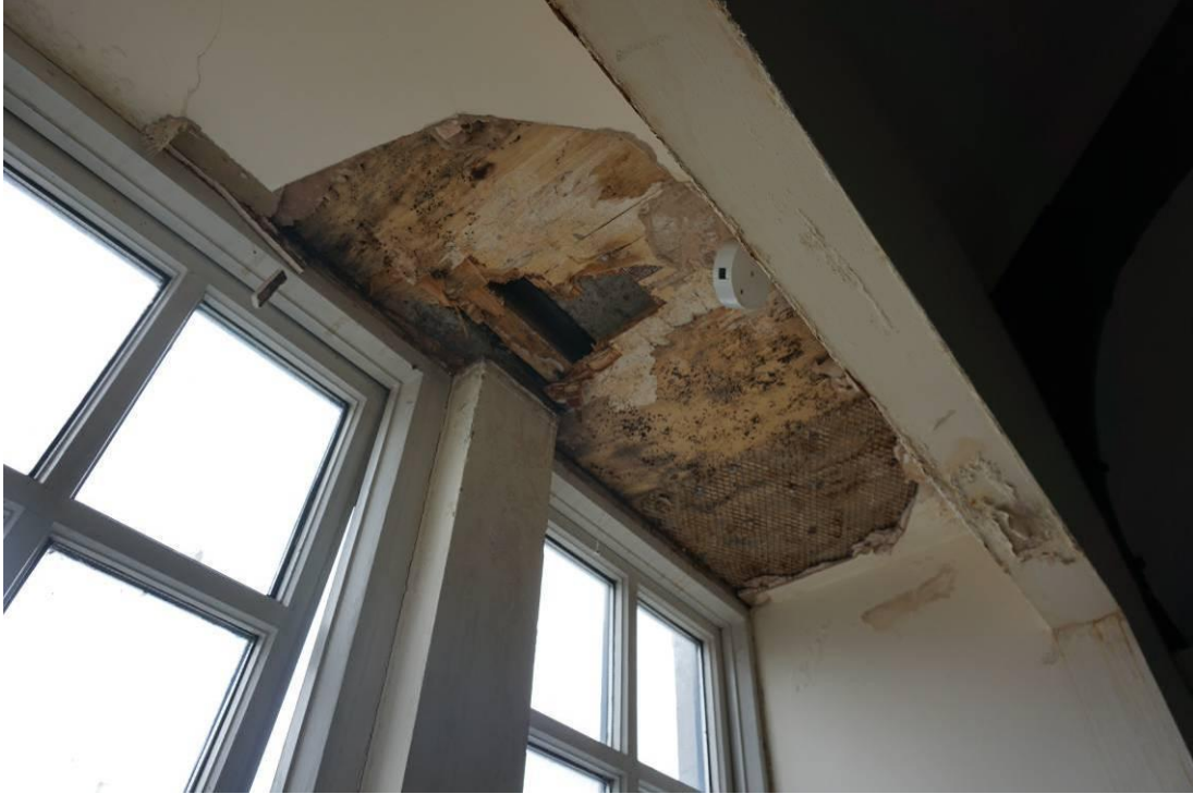
Photograph 2 Window head soffit with water ingress damage. Note DPC detail, poorly installed.
