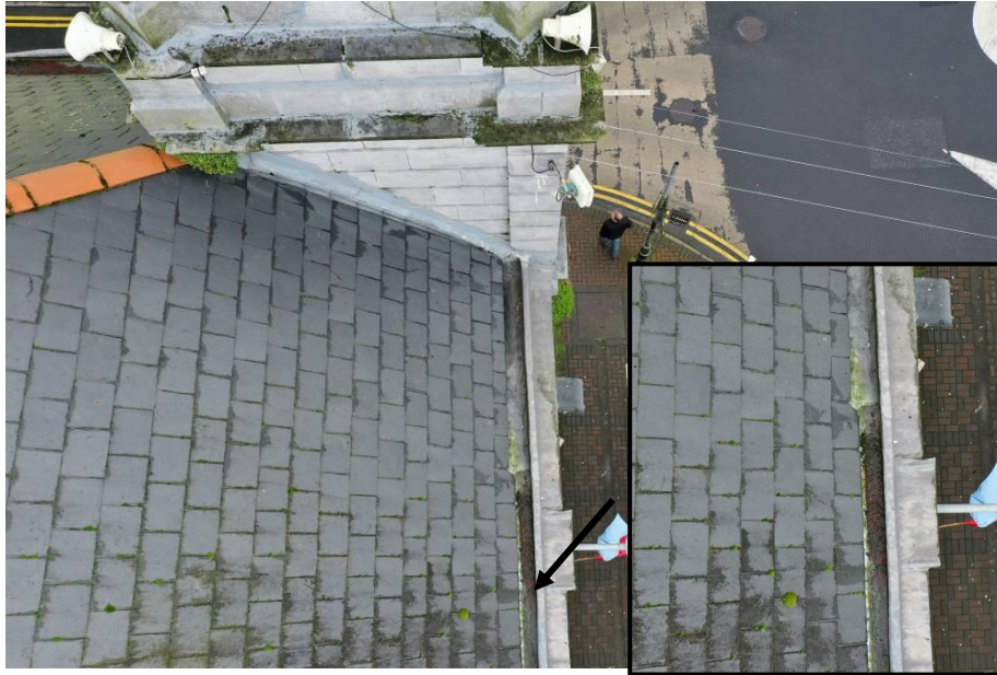
Photograph 11 View of problematic area of the parapet gutter (North, by tower). Note signs of poor fall and water pooling (Highlighted). This area requires attention.
