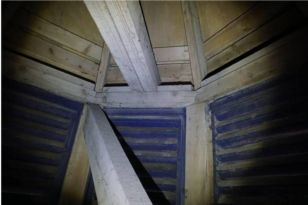
Photograph 3 Internal view of the Louvre panels.
