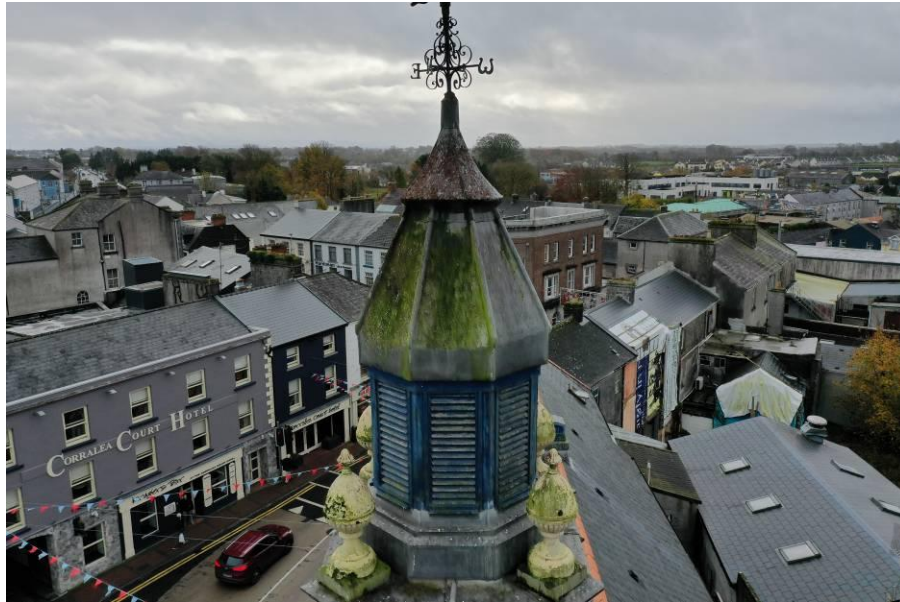
Photograph 7 Section of the RLS roof, heavily stained in bird guano.
