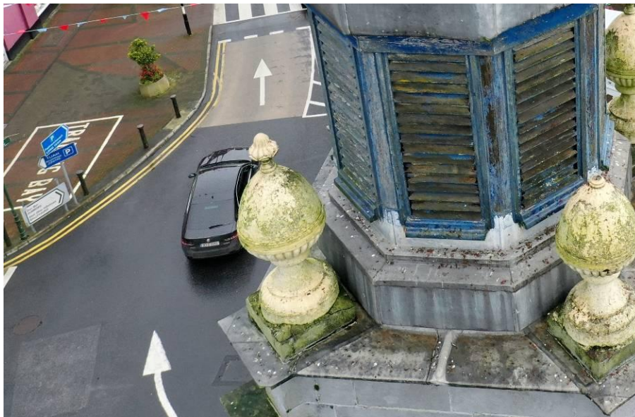
Photograph 8 Detail of “Urn” on the upper ledges. Note cracking to concrete surround.
