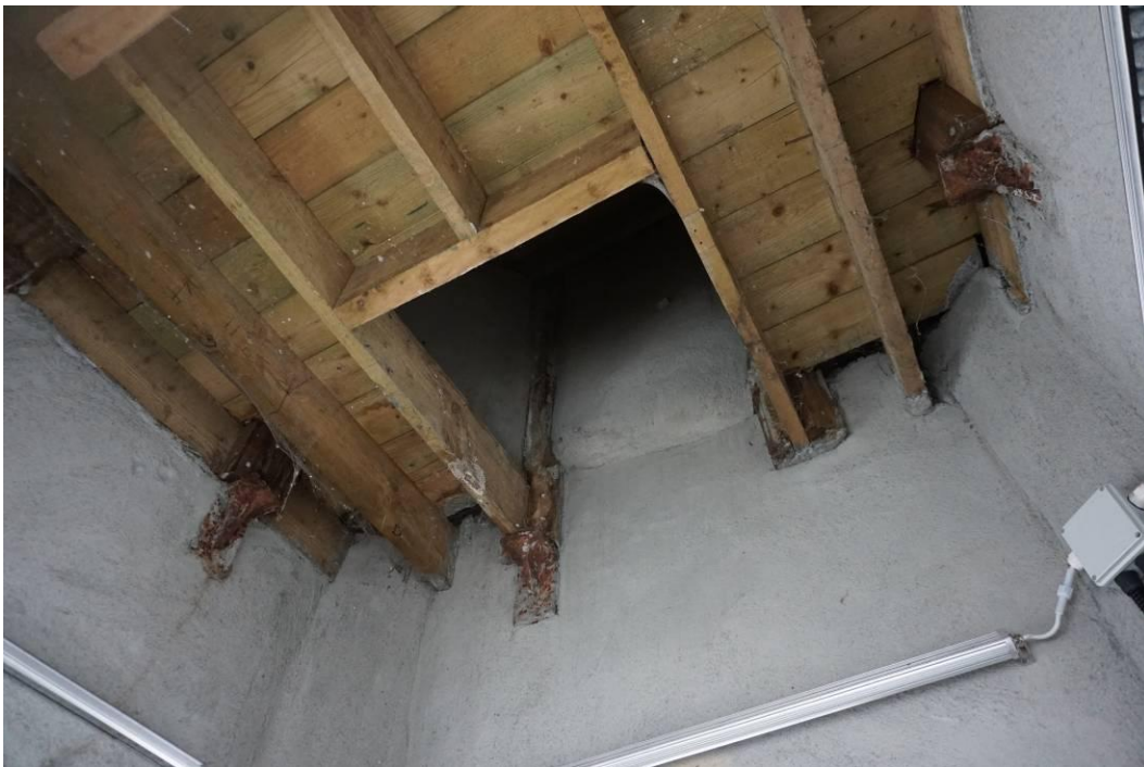
Photograph 5 View of underside of upper floor deck. Note supports with cementitious render applied around them. These supports are either mechanically fixed or built into the fabric.
