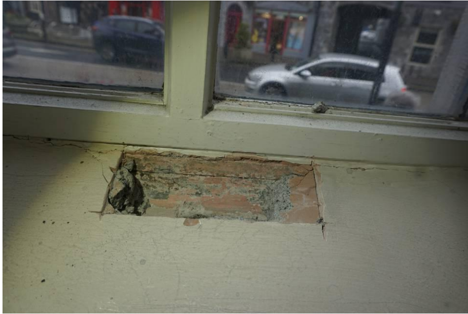
Photograph 39 View of investigative opening up at the window frame, top of window cill splay.
