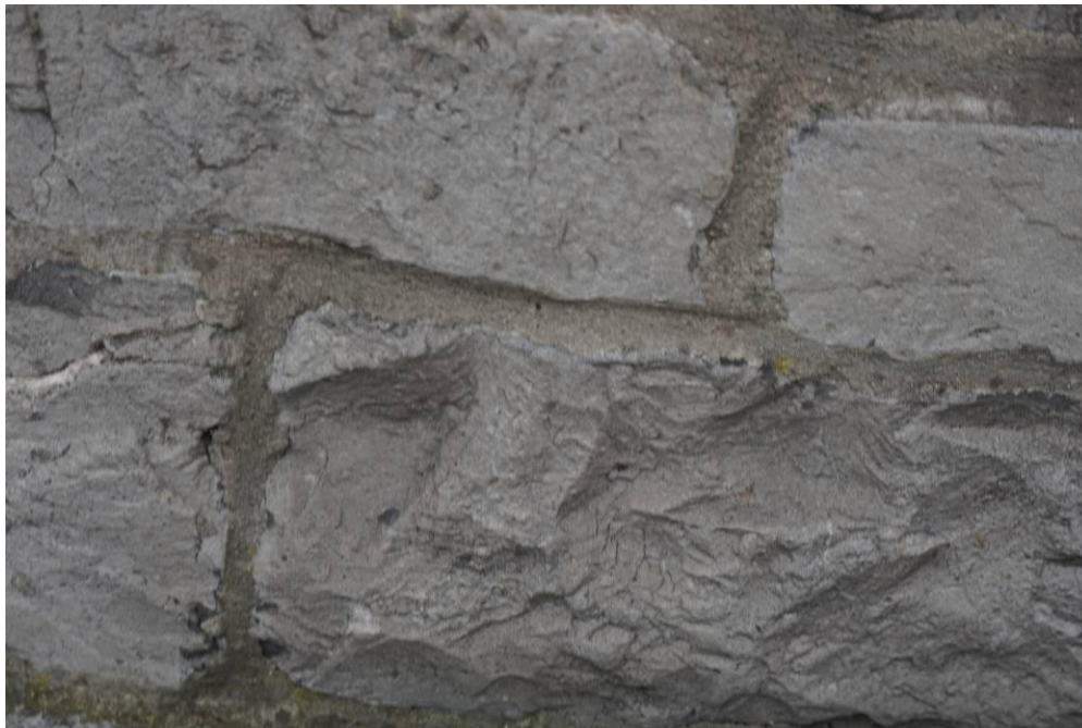
Photograph 16 Detail of the cementitious mortar pointing.
