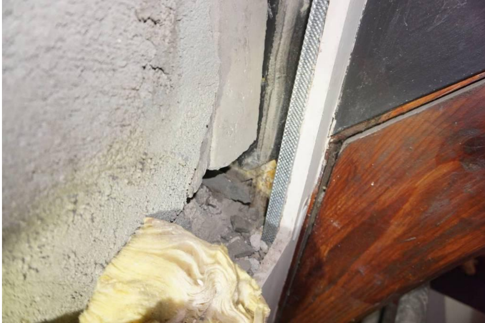
Photograph 33 View of the truss where fitted against the masonry.
