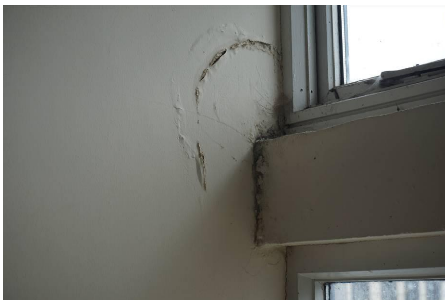
Photograph 19 Detail of centre mullion. Note signs of water ingress on window jamb.
