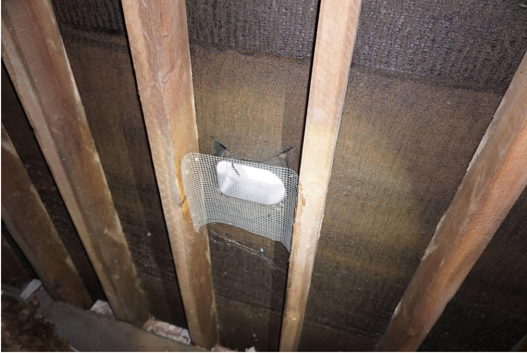
Photograph 29 Mesh applied across one of the vents.
