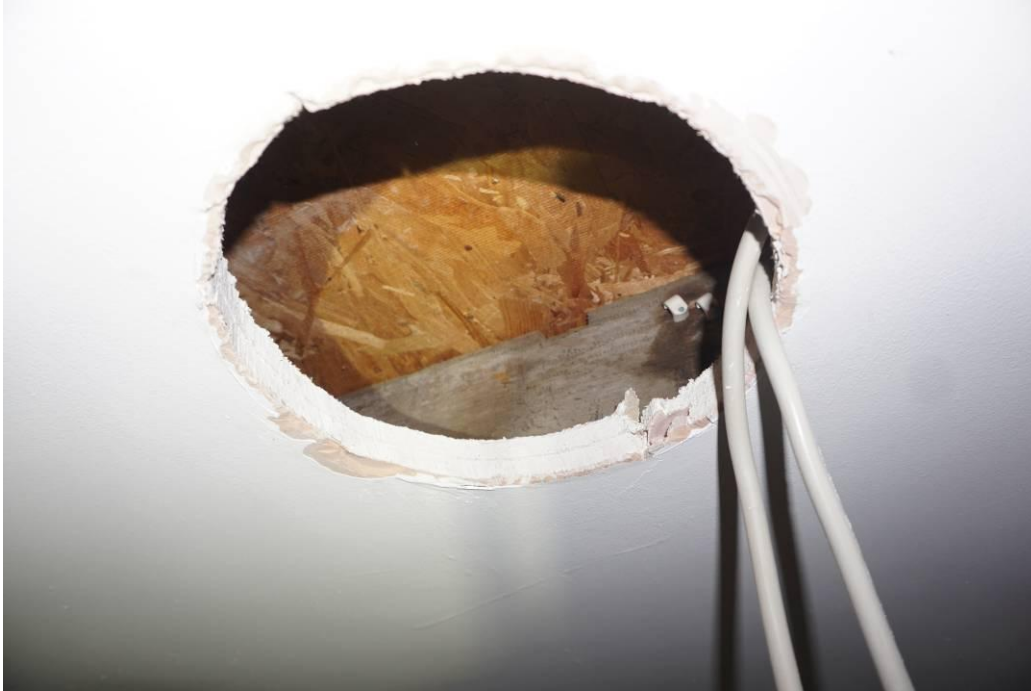
Photograph 35 Penetration for the light fitting.
