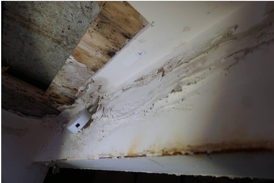
Photograph 25 Fabric damage from water ingress.
