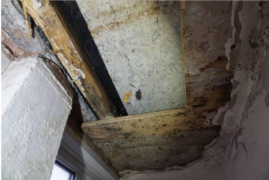
Photograph 24 Detail of the opening up works to the window head.
