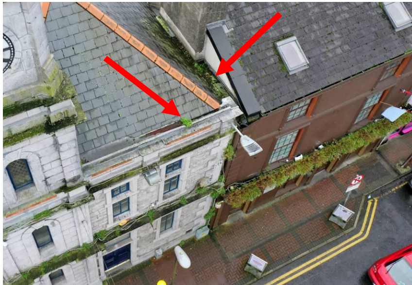
Photograph 10 View to end elevation of Tuam Town hall. Note block parapet gutter and heavy vegetation to abutment gutter of neighbouring property (Highlighted).
