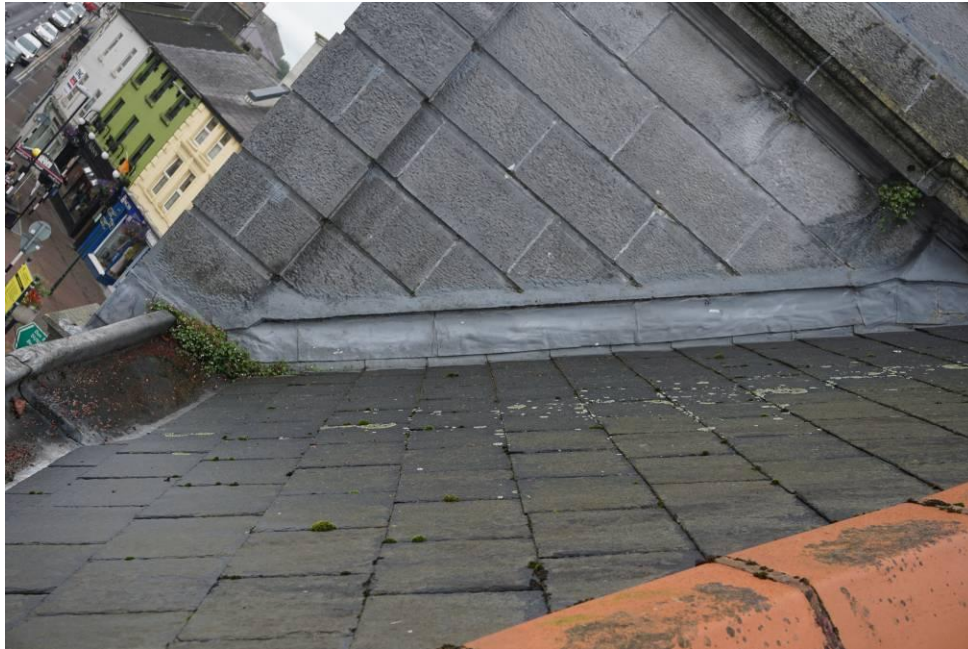
Photograph 17 View of flashing detail to the tower.
