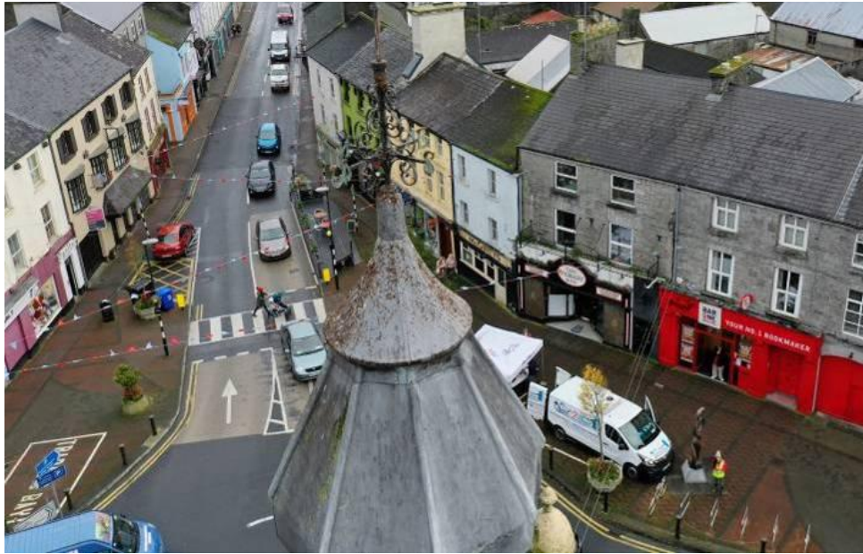
Photograph 6 Top section of the tower, covered in Rolled Lead Sheet.
