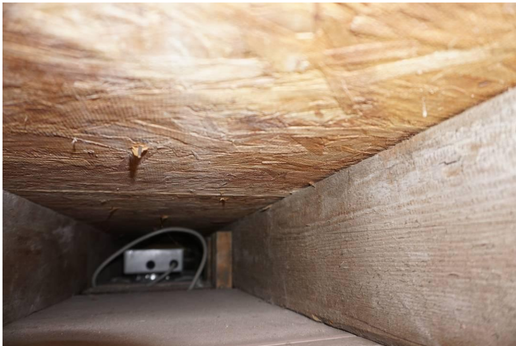
Photograph 36 View of junction box within ceiling void.
