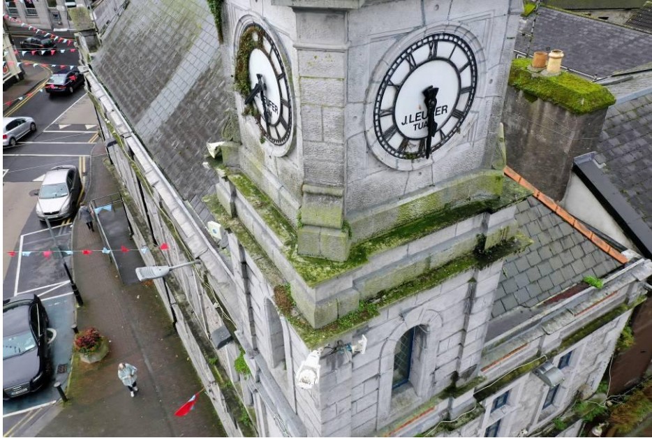
Photograph 9 Mid section of the tower. Masonry pointed with mastic. Heavy vegetation growth and staining.
