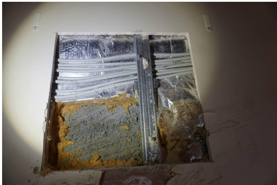
Photograph 23 Detail of the panel. Note adherence of the fiberglass to the render.
