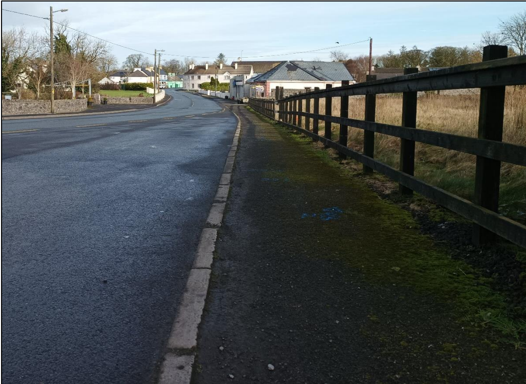
Photograph 2.2: View North of Existing East Side Footway
