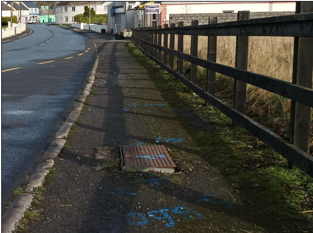
Photograph 2.6: Utility Manhole Cover on East Side Footway
