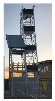
At the rear of the fire station there is a training tower. This is a steel framed structure fixed to a concrete base, similar to the one in the photo,
