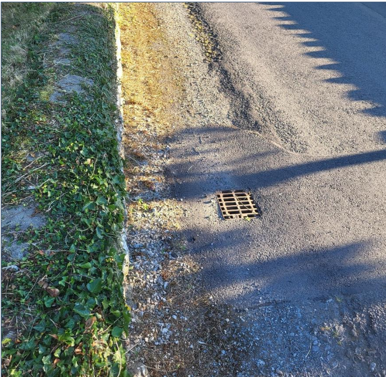
Plate 2-4 Storm drain, adjacent to the western boundary, buffered from the sit by the block stone wall.
