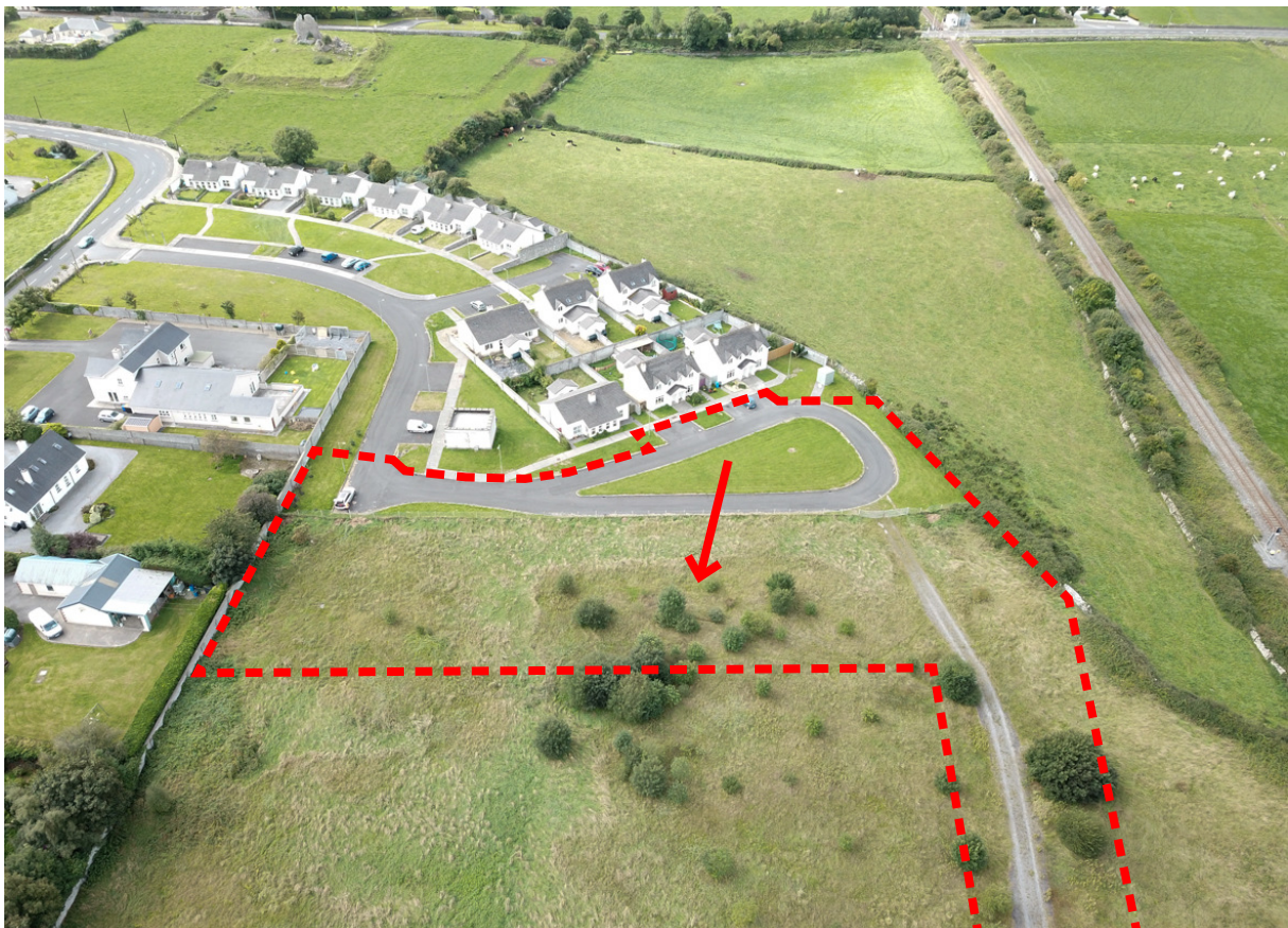
Fig 1.1 Proposed site outlined in red. Position of photograph in Fig. 2.1 indicated with red arrow.
