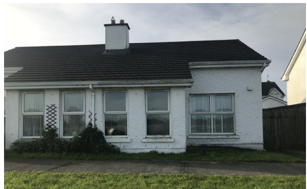
D. 1-Storey semi-detached houses opposite proposed site.
