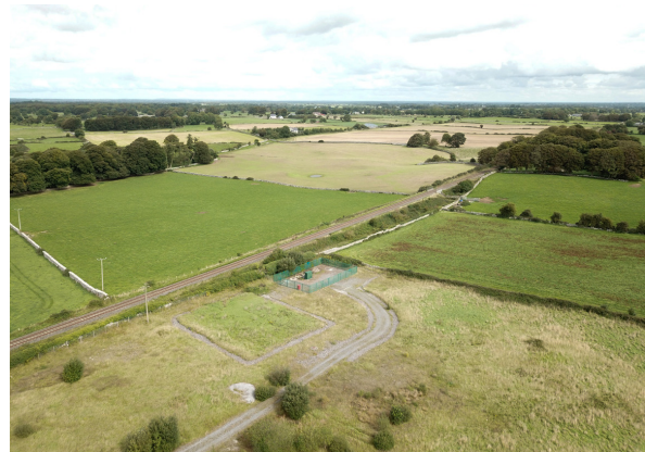
Fig 2.3 Wastewater treatment facility to the rear of the site.
