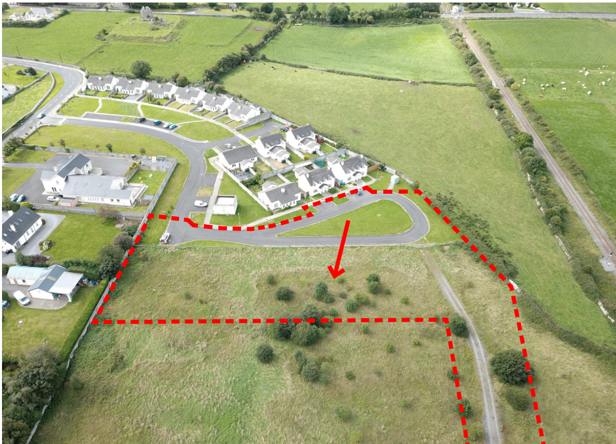
Fig 1.1 Proposed site outlined in red. Position of photograph in Fig. 2.1 indicated with red arrow.
