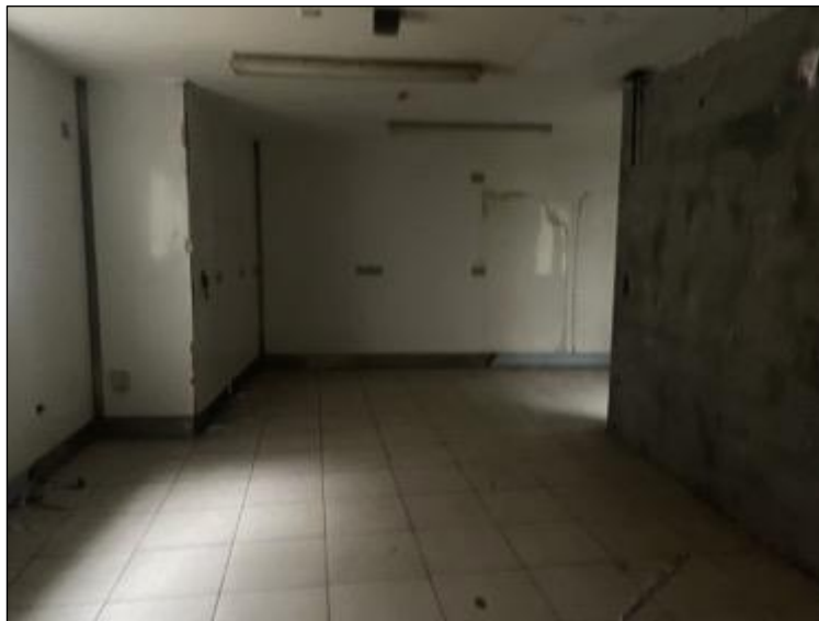
Plate 5: Former kitchen/food preparation area. Taken from S.
