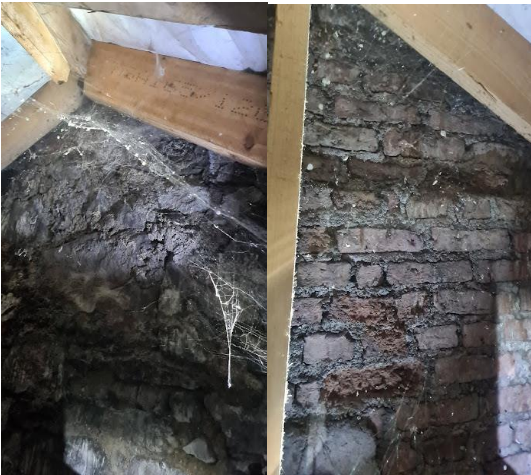
Plate 3-6 Southern gable wall
