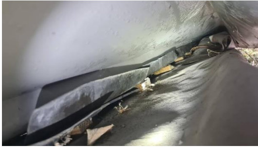
Plate 3-8 view under bitumen
