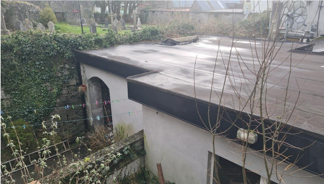
Plate 3-3 Bitumen felt roof with potential access
