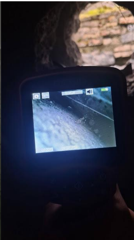
Plate 3-11 Inside wall cavity
