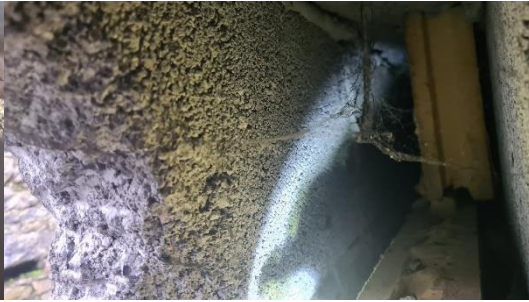
Plate 3-9 Inside cavity wall
