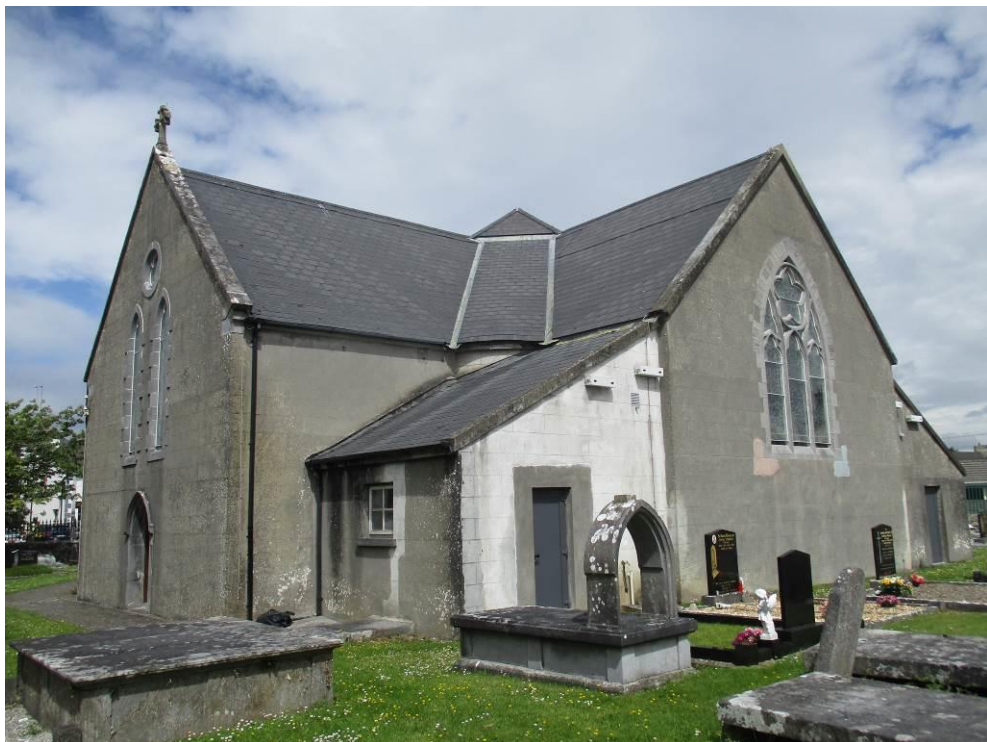
Image 5. IMG_0521. Building Southwest view.
