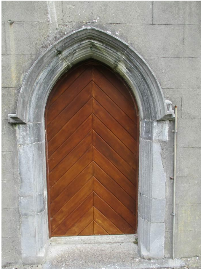
Image 6. IMG_0530. Exit door. South Elevation.
