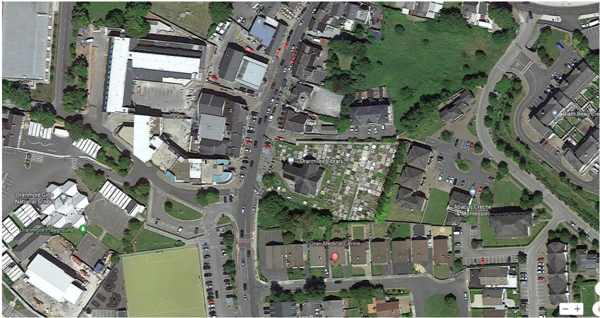
5. Present day aerial view of Oranmore Library Building and surrounds.
