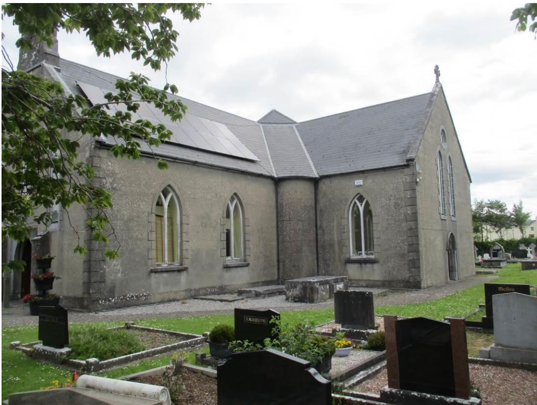
Image 1. IMG_0506. Building South Elevation view.
