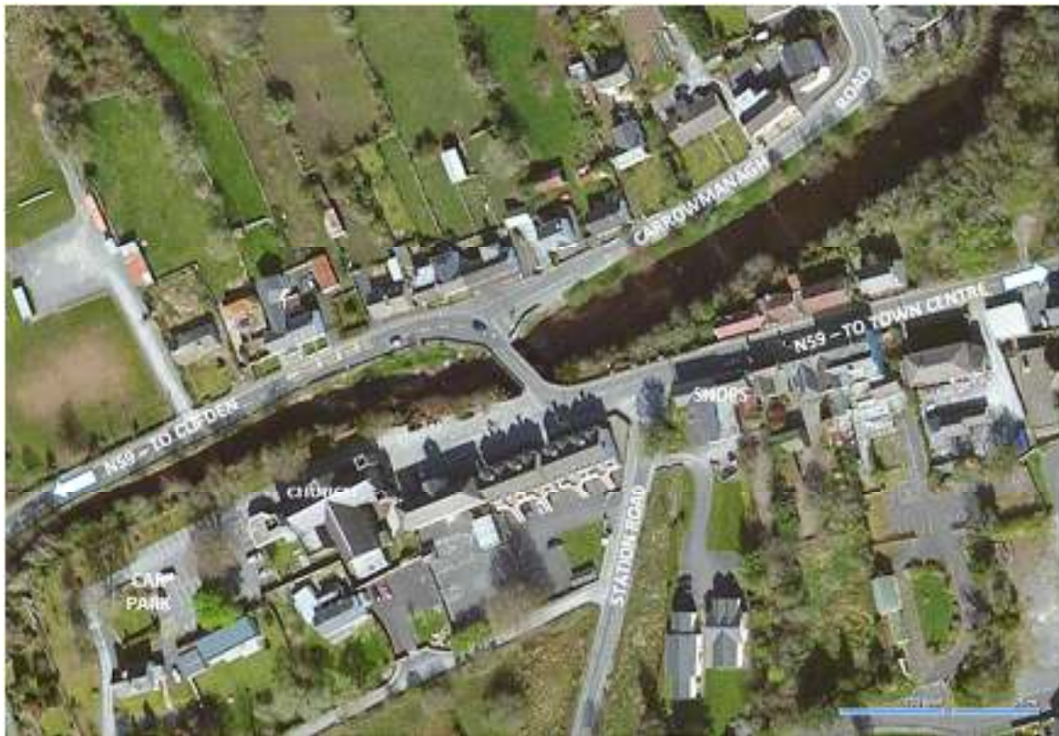
Figure 1.1. Aerial image of Oughterard Bridge
