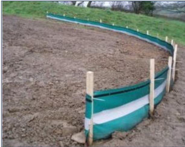
Plate 3-4 Embedded Silt Fence
