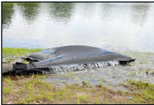
Plate 3-1 Silt Bag with water being pumped through.
