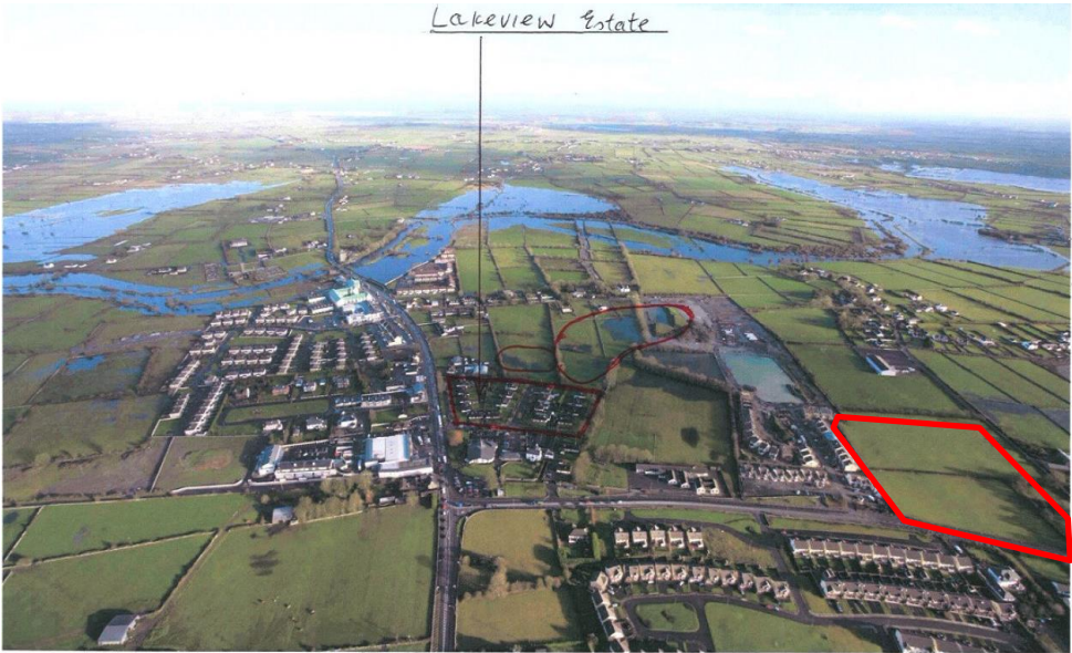
Figure 3-2 Lakeview flooding December 2006
