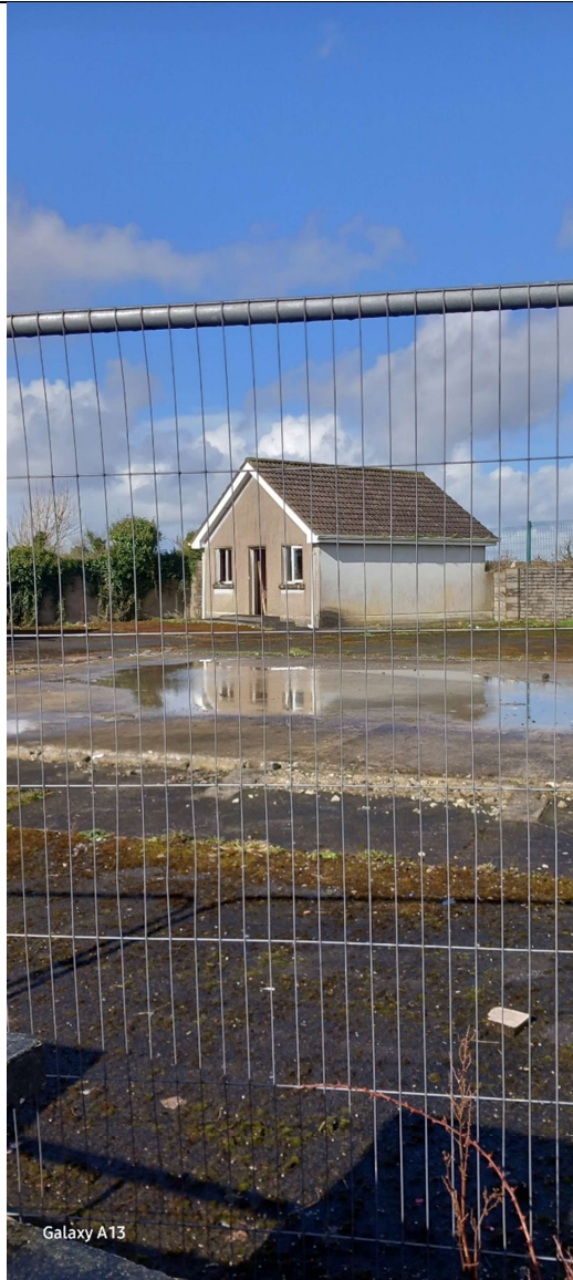
Figure 3.5 - Existing Shed (Retention is sought for in this planning application)
