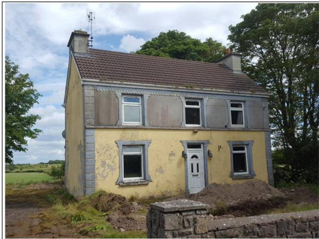
Photograph 2: Front Elevation of The Existing Dwelling taken from within the site
