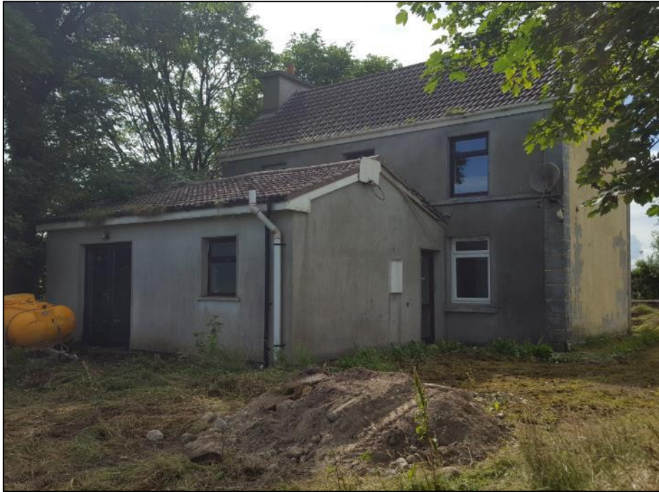
Photographs 3: Photograph taken from within the site
