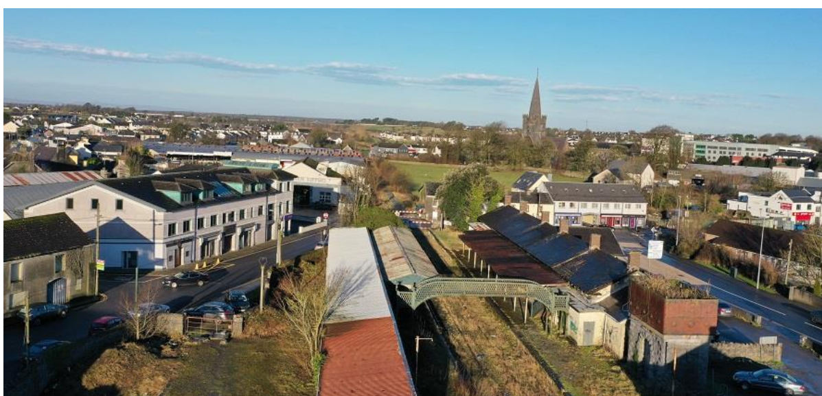
Figure 2: Station House building in context
