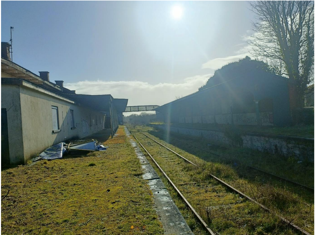
Plate 5: railway track at station
