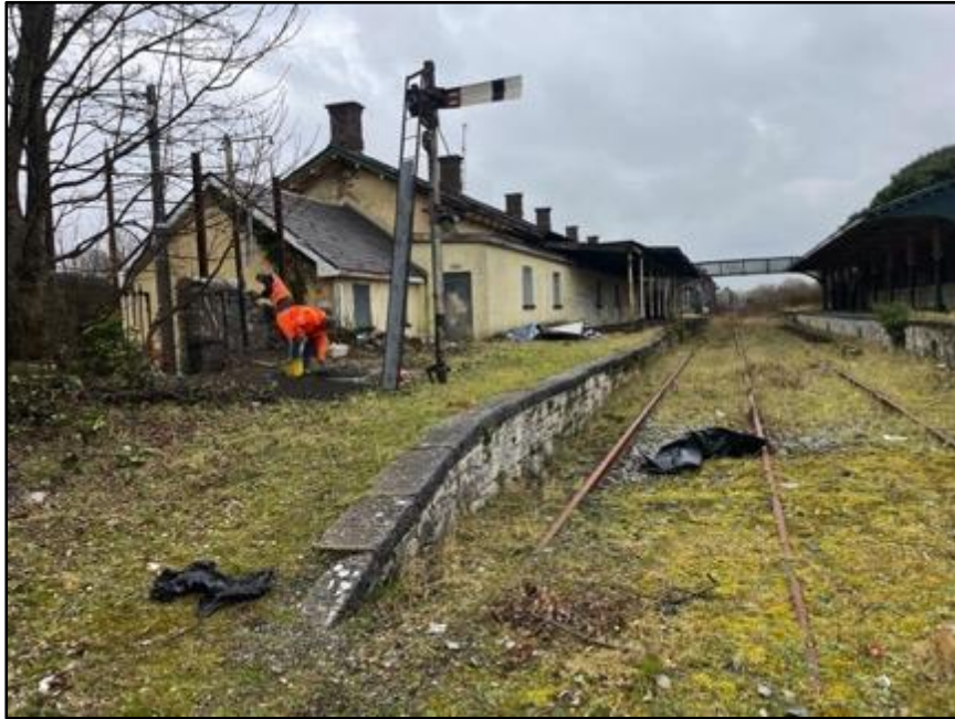
Plate 3: View of railway building, platform and track from the NW.
