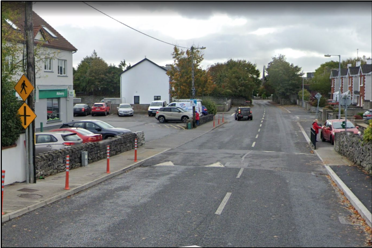
Figure 3.8: Raised pedestrian crossing on the Tuam Road, R347 with signage, tactile paving, railings and reflective bollards. This crossing to the local store is 160m from the Cullairbaun entrance. (Source: Google Street View)
