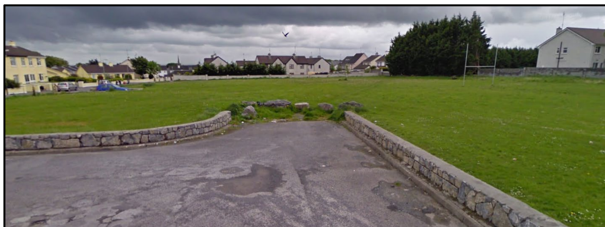
Figure 3.2: Provision made for access to the site located in the Cullairbaun Estate (Courtesy: Google Earth, Street View)
