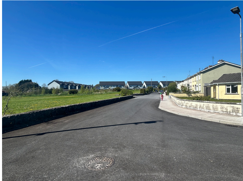
View of proposed development site, looking north west from existing Cullairbaun estate (PKA)
