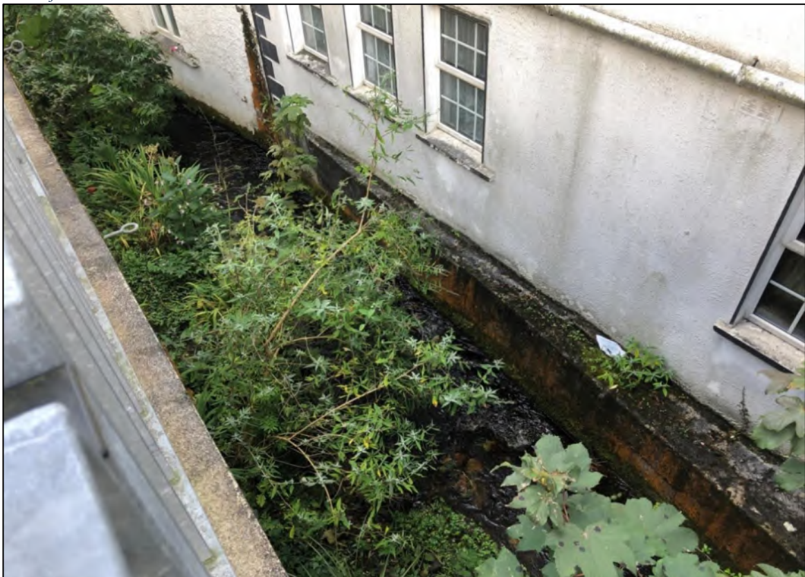
Plate 3-8 An artificially canalised section of an unmapped EPA watercourse, classified as an Eroding Upland River (FW1) runs culverted under Main Street in Clifden Town Centre to the northeast parcel of the proposed works site. This artificially canalised watercourse continues to flow adjacent to the eastern margin of the proposed works site, in a southerly direction before discharging into the Owenglin River after approx 280m, which at this point is designated as part of the Twelve Bens/Garraun Complex SAC
