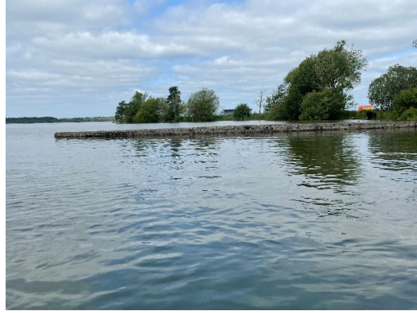
Plate 10: View from slipway at south-eastern corner of site facing northwest
