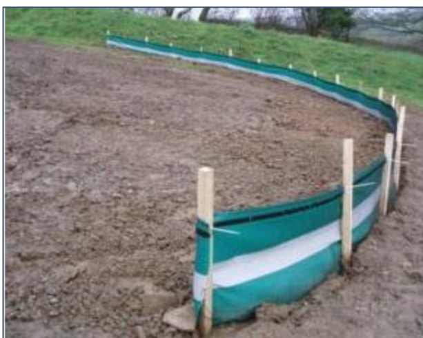
Plate 3-4 Embedded Silt Fence
