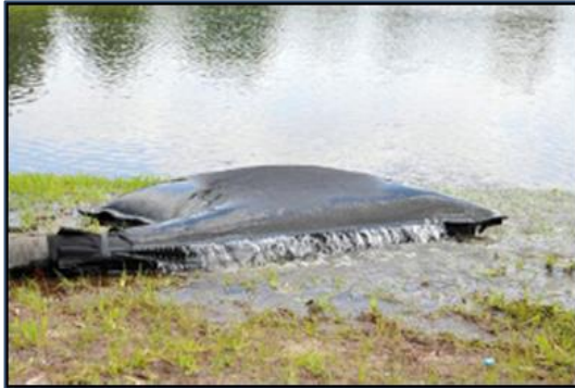
Plate 3-1 Silt Bag with water being pumped through.
