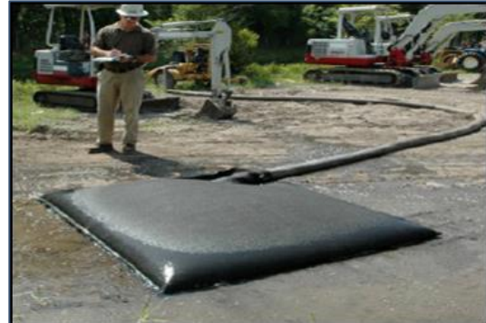
Plate 3-2 Silt Bag under inspection
