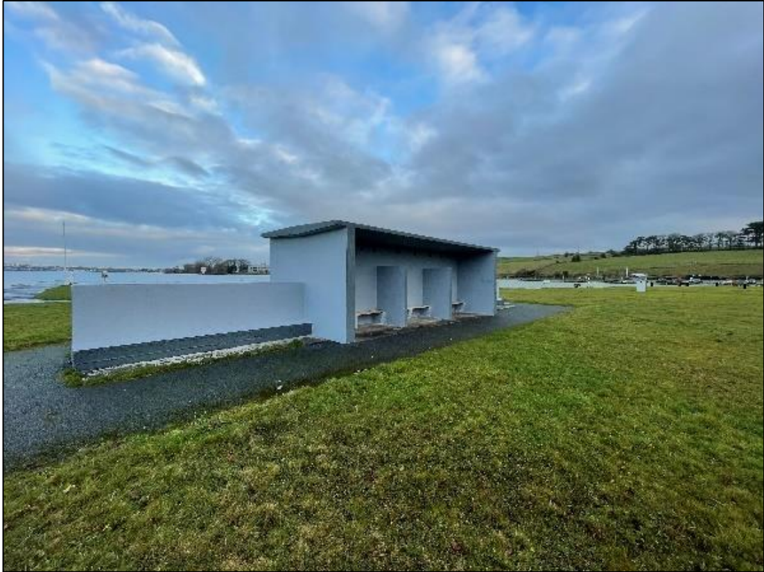
Plate 5-6 Existing changing shelter to be demolished within the Proposed Development site.
