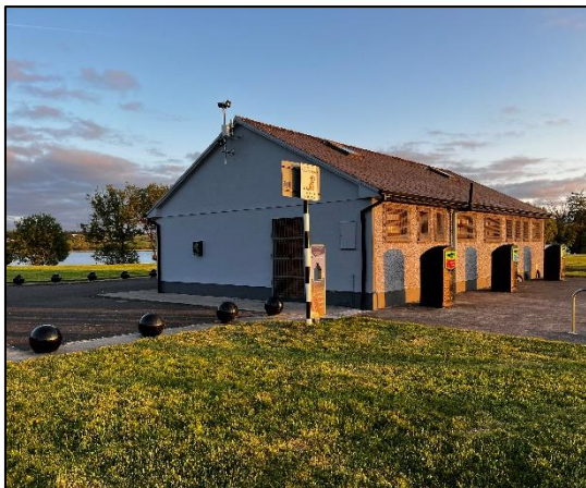
Plate 5-10 Existing toilet block which was assessed as a potential PRF.
