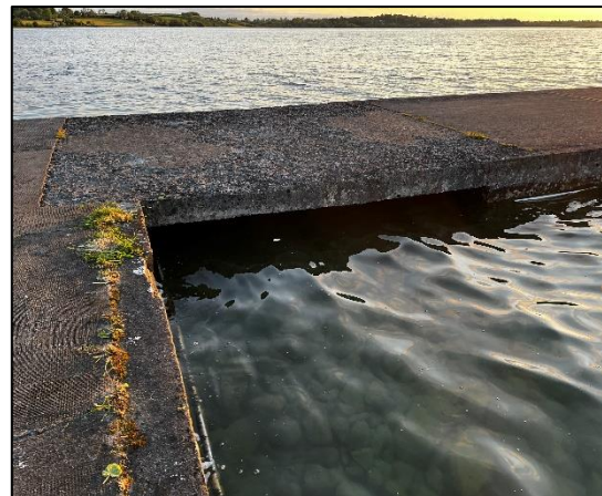
Plate 5-11 Example of a pier within the Proposed Development site.
