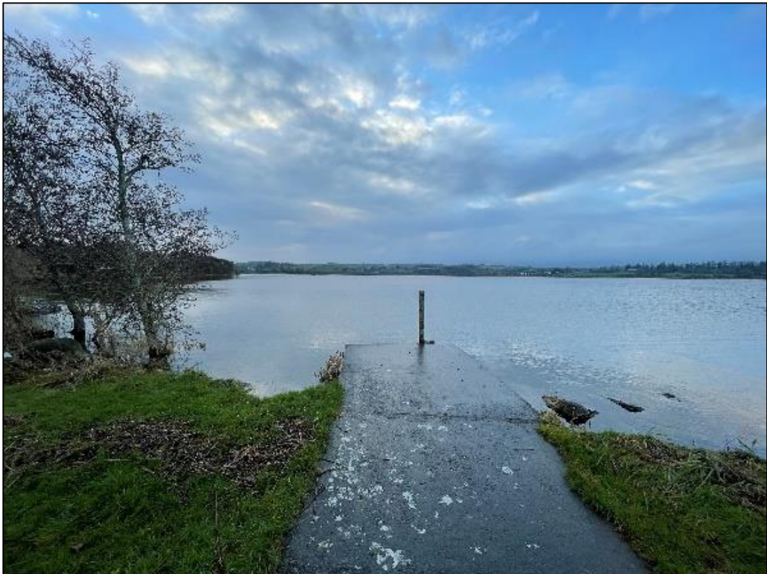
Plate 5-7 Existing slip into Lough Rea which will be upgraded.
