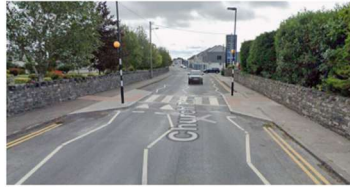
Figure: Screen grab from Google Street view showing the current zebra crossing with hostile projections into the live traffic lane.
